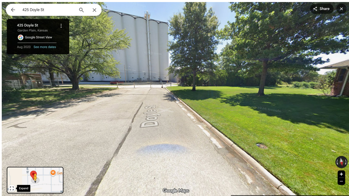
Southern view from N. Doyle St. to Co-Op (dead-end street)
