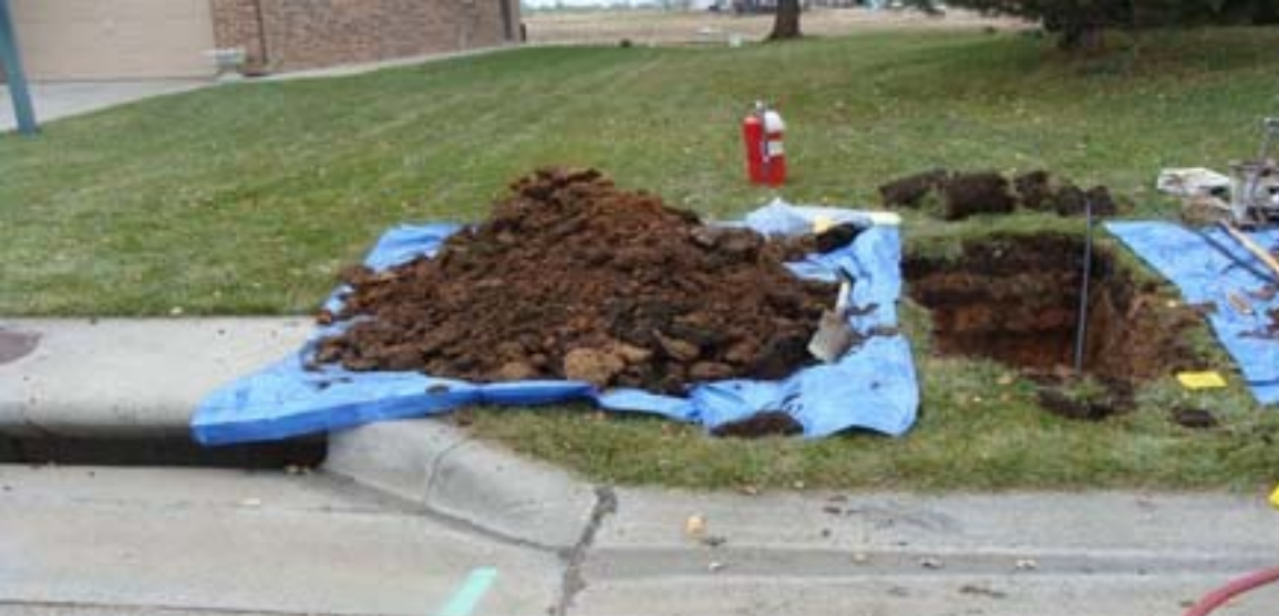
Boring under the street and installing gas service to new homes
