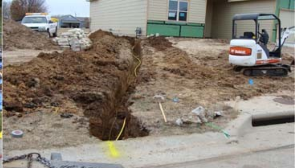
Boring under the street and installing gas service to new homes
